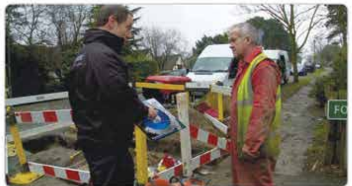
Service & support on site
